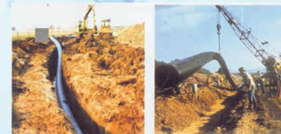
*Picture 2.1.5- Making connection out of the trench and laying down the pipe.*
