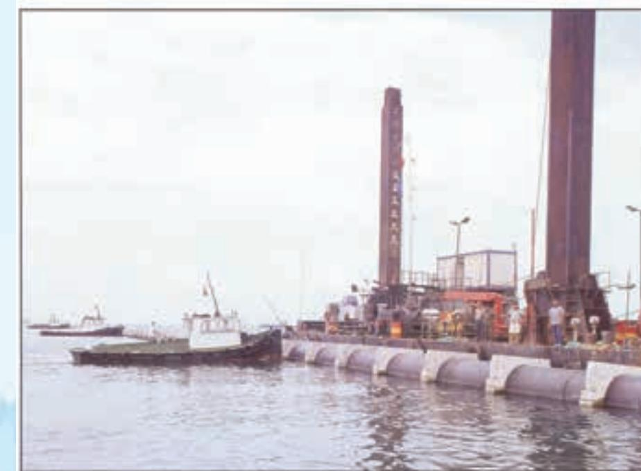
**Picture 2.1.7a-** A view from sea discharge application of 1600mm PN 4 PE pipes.
